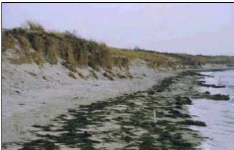
Fig. 8: Lee-side erosion and filter tube system at Køge Bay.
