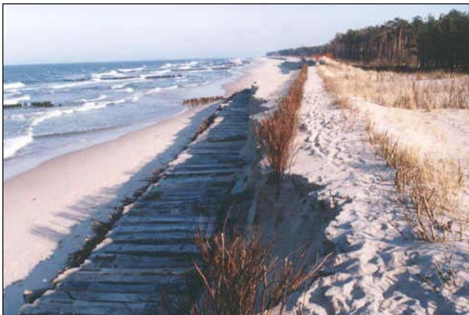
*Fig. 20: Structure of combined seawall visible after strong erosion of the protected dune, Władysławowo Harbour, 1995 (photo by K.Furmanczyk).*
