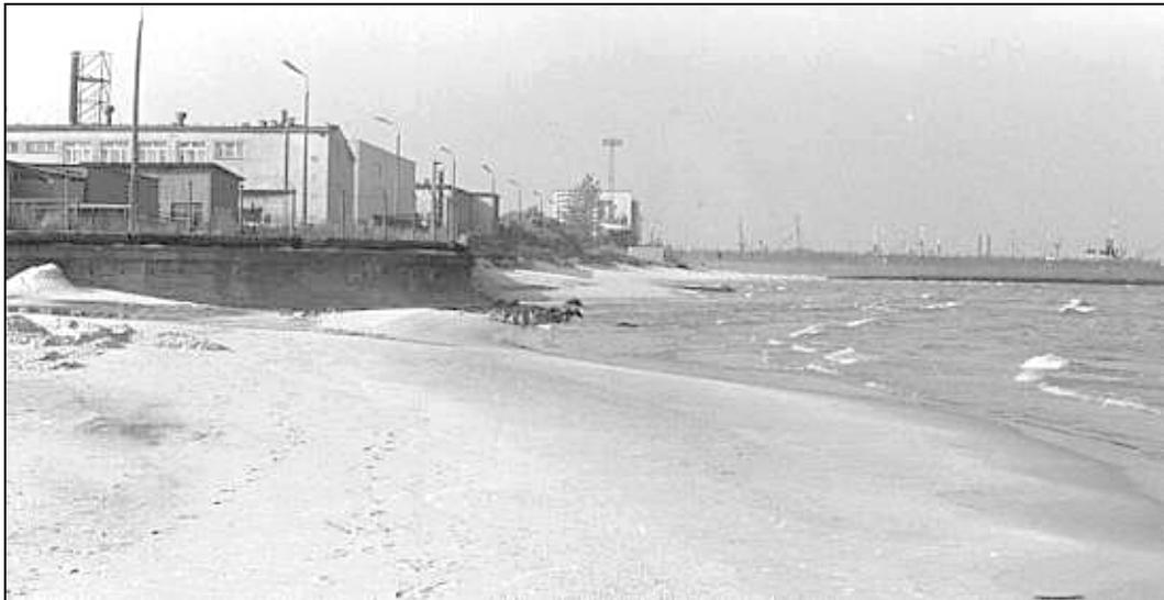
*Fig. 26: Hard concrete seawall on the east from Wladyslawowo Harbour, 1991 (photo by K.Furmanczyk).*
