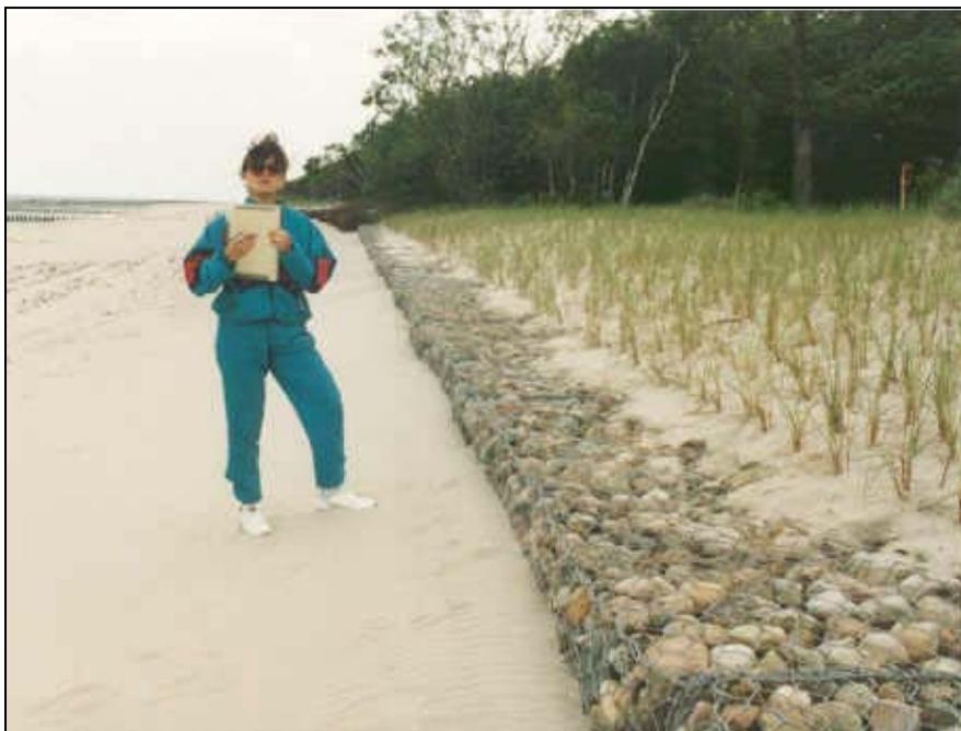
*Fig. 24: Medium seawall, slope behind the seawall revegetated, region of 8 km, 1994 (photo by K.Furmanczyk).*
