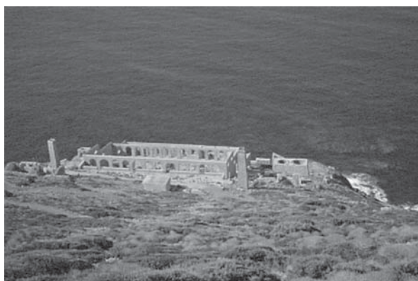
Fig. 4. On the steep coast underneath the town of Nebida the Lamarmora washery is situated, which treated the minerals of the Nebida mine. It represents one of the most interesting mine-archaeological sites of this part of the coast.
