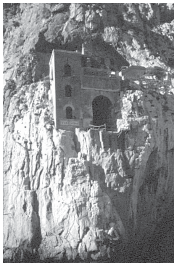
Fig. 3. The archaeological mine site of Porto Flavia, a subterranean tunnel constructed in 1924, ending at 36 m height on a limestone cliff above the sea, enabling to load the ships with Pb-Zn minerals exploited in the Masua mine, reducing in this way shipping expenses significantly.
